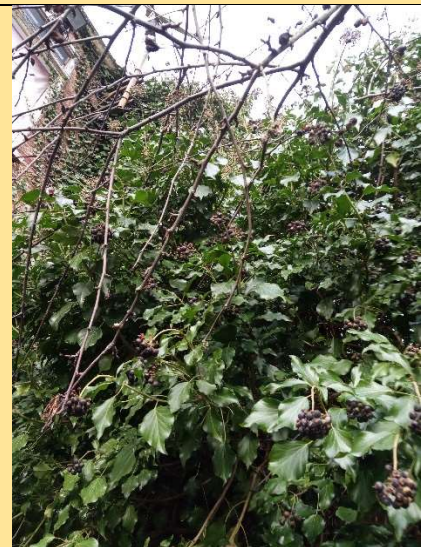
Foliage at back had to be cleared so that boiler flue can be fitted
