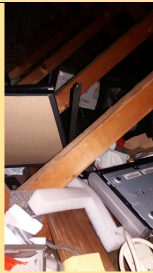
Loft needed clearing before insulation could be fitted
